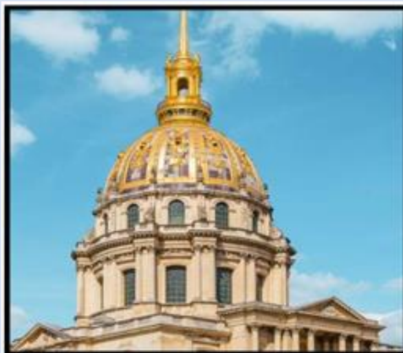
Figure 1B: Gold roof of Les Invalides (Paris France): The gold dome forms the roof of Napoleon Bonoparte's final resting place in France; The gold retains its shine and does not oxidise when exposed to the atmosphere.
