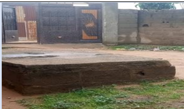
Plate 6: A typical soak away at Angwan matta.
