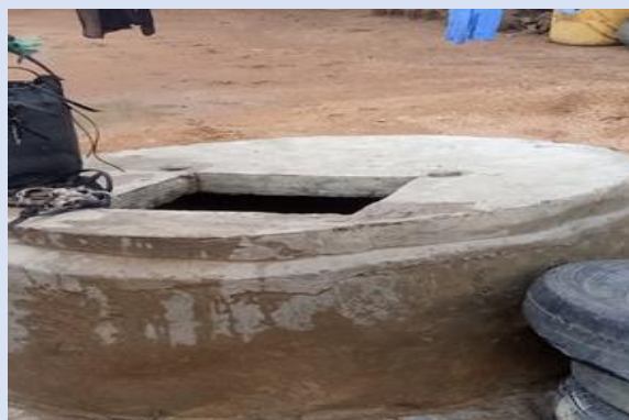
Plate 3: Cemented shallow well at Angwan gate.
